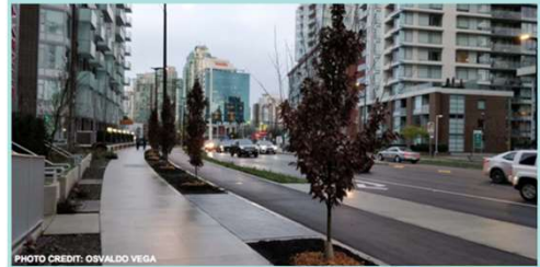
Case study: Rainwater tree trenches at Quebec Street and 1 st Avenue, Vancouver
